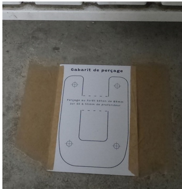
Template secured in configuration 1.
